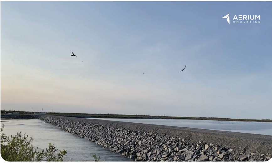
RoBird chasing birds during the Weir reconstruction project in Churchill, Manitoba.
